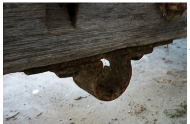
Figure 16 – Axletree Bands fitted to the Warrnambool Casemate Gun Author's Photograph (©2016)
