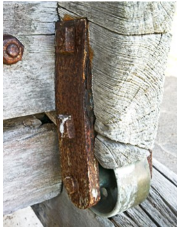
Figure 11 – Front Carriage Roller fitted to the Warrnambool Casemate Gun Author's Photograph (©2016)
